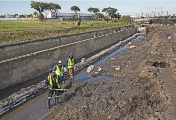
Building back better: City teams are in the home stretch of the structural rehabilitation of a section of the Blomvlei canal wall in Belgravia.
